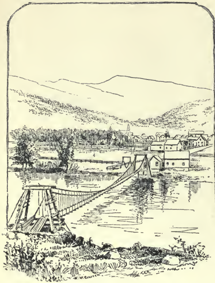
SUSPENSION BRIDGE, GORHAM, N.H.
